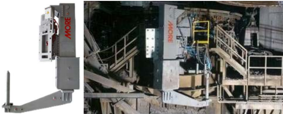
Fig. 13 – STROP in operation on the EAF in Mexico
