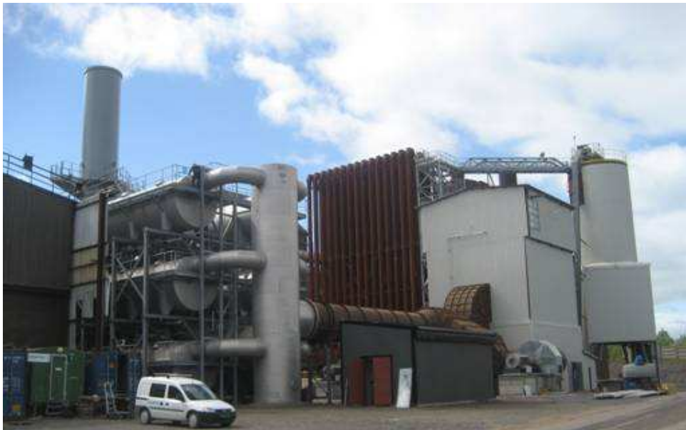
Figure 5: the new primary fume treatment plant.
