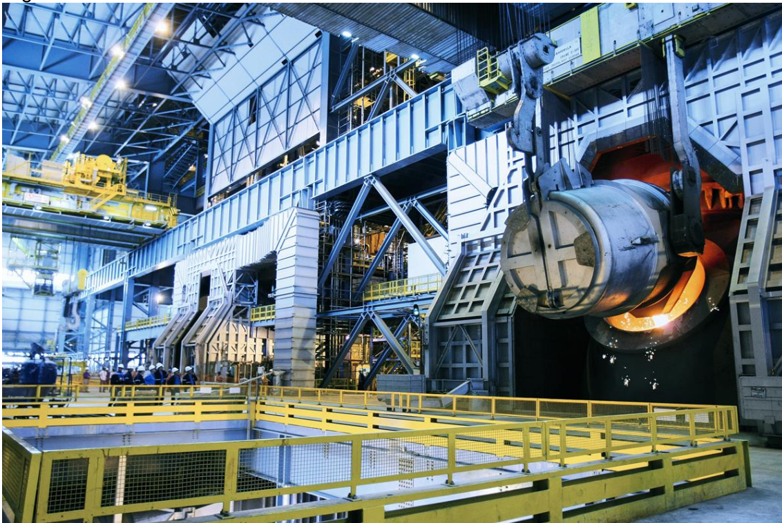
Figure 1: tkCSA converter (330 ton)
