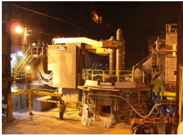
Figure 2. Engineering View and Actual View at slag door side 1.
