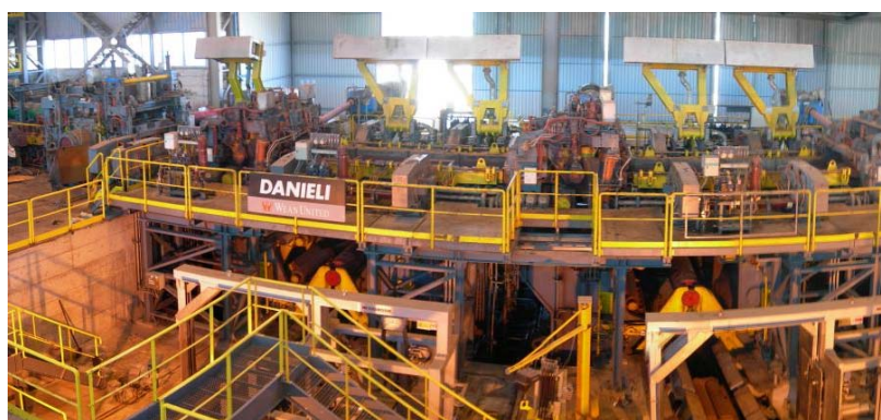
Figure 7: High-speed shear and high-speed downcoiler area
