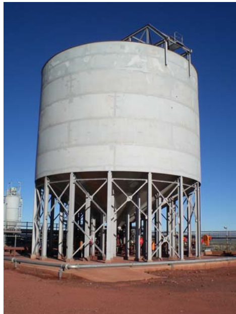
Figure 9: 18 m diameter WesTech Deep Bed™ paste thickener
