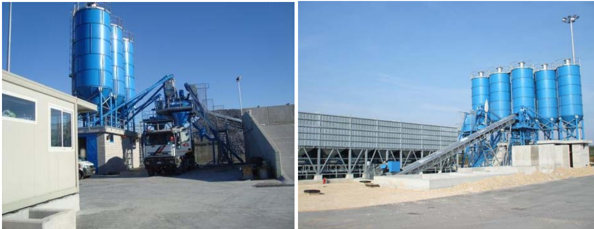
Figure 11. The A.B.S. concrete plant in Italy, that utilize slag in the concrete like aggregate.
