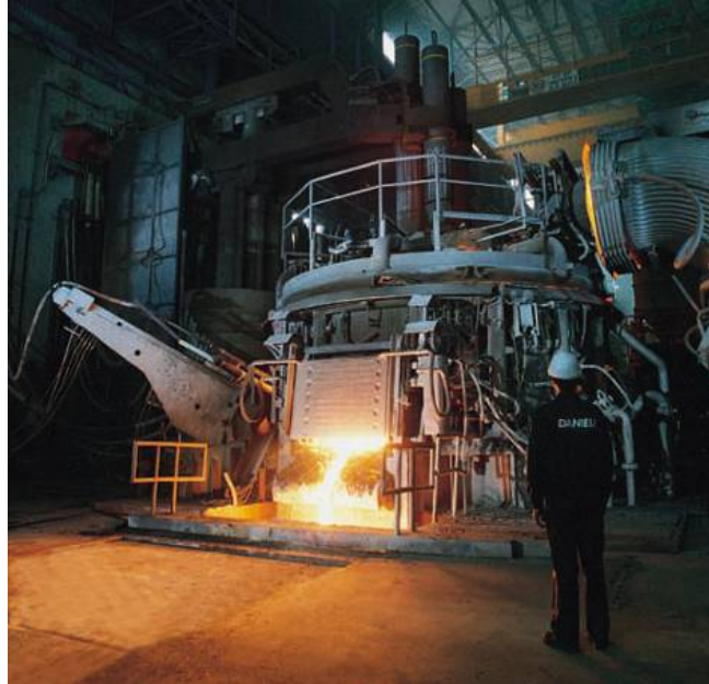
Figure 1. Danieli Electric Arc Furnace .
