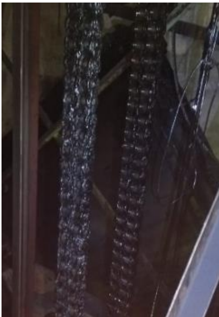
Figure 5. Detail of the counterweight drop
