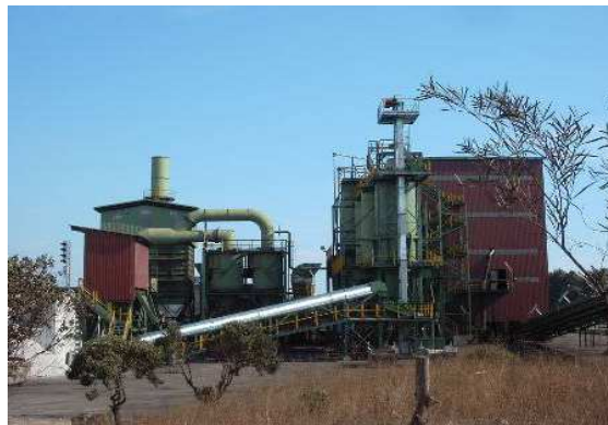
Figure 4: Briquetting plant, ILVA Taranto, Italy
