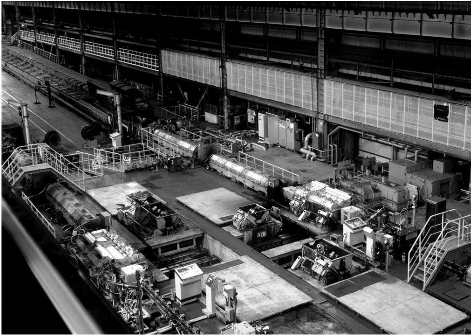
Figure 9 – Reducing/Sizing Mill and Water Box Installation
