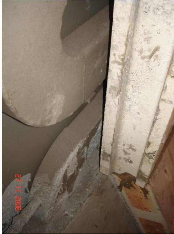
Figure 10: Security lining casting.
