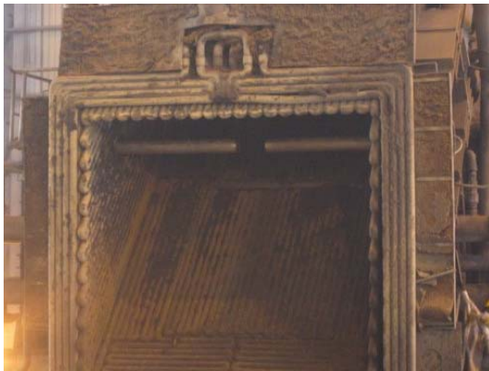
Figure 7. The installed lances
