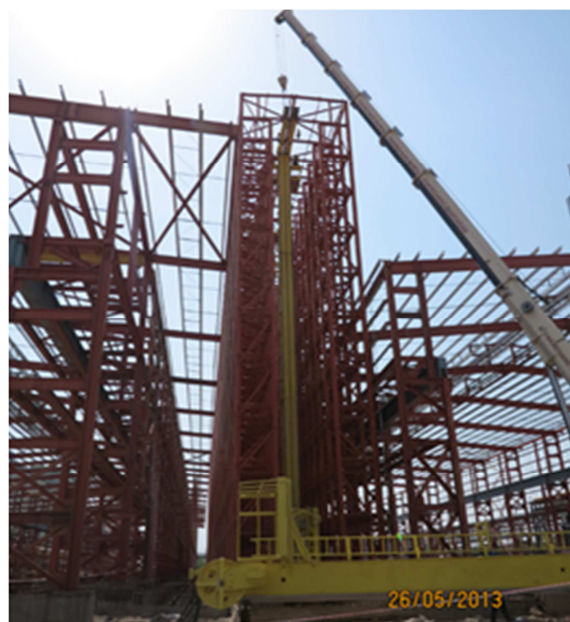
Figure 19: Rack supported warehouse in JSW
