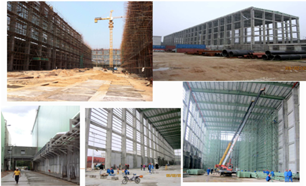
Figure 16: Typical free standing rack constructions
