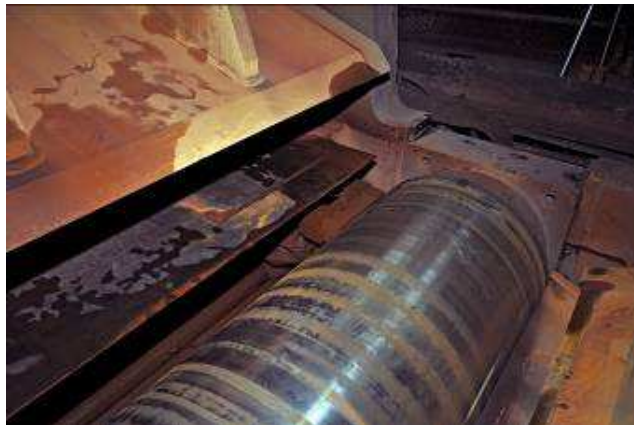
Figure 10: Pinch-roll polisher installed at voestalpine Stahl, Austria
