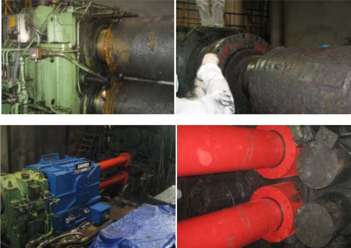
Figure 16. Before and after gear spindle replacement on HSM F7 finishing stand.
