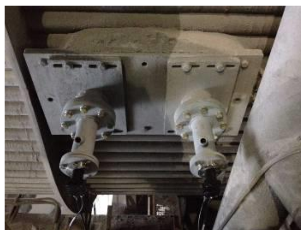
Figure 9: Installation of OVM at SDI
