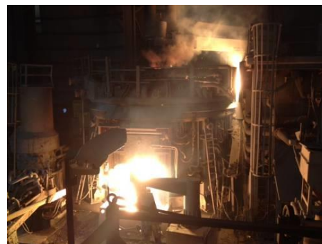
Figure 11: As installed at SDI
