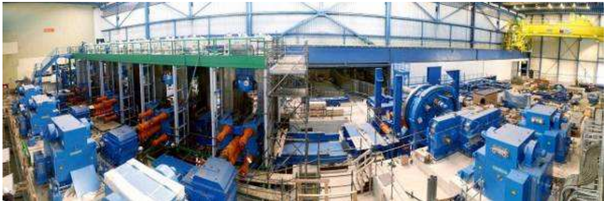
Figure 1: CM22 during assembly at Corus IJmuiden, Netherlands.
