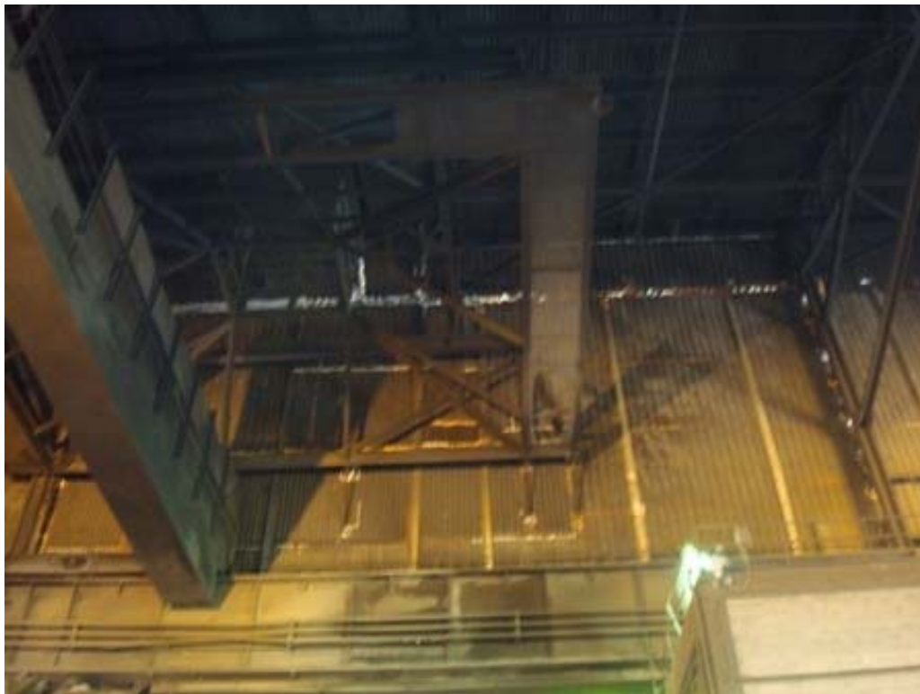
Figure 17. Existing sheeting sealed with high temperature sealant.
