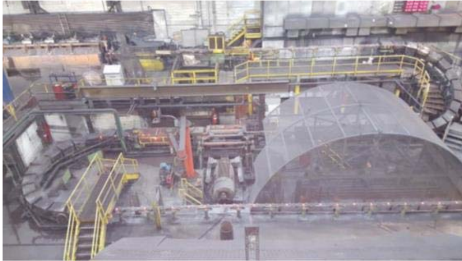
Figure 11. Pre-finishing mill area after modification.
