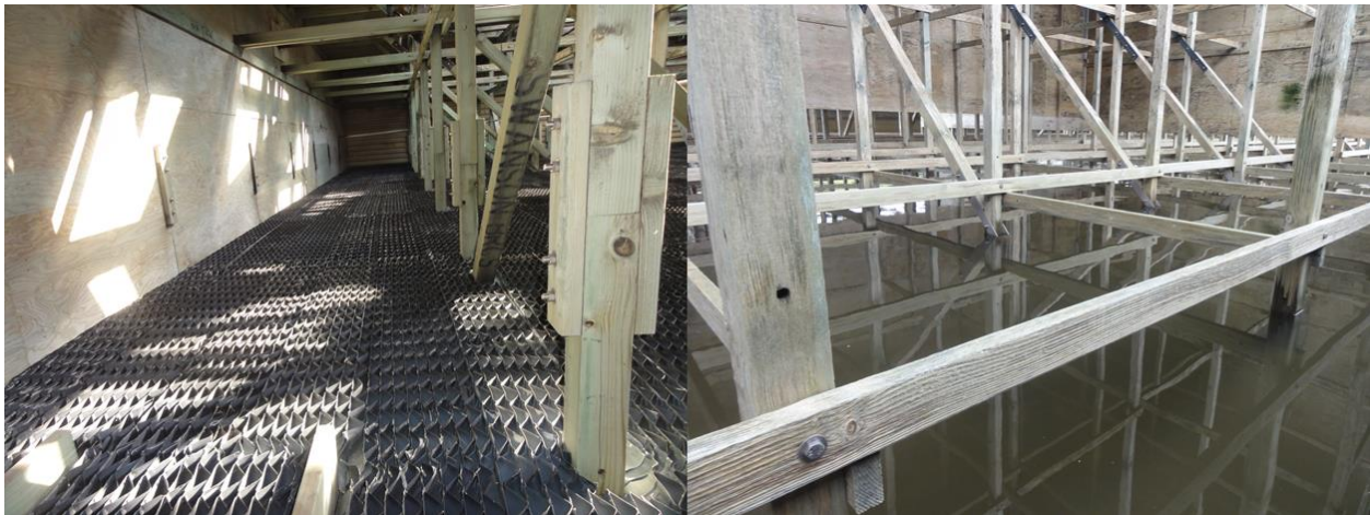
Figure 10 – Cooling tower inspected in September 2015.
