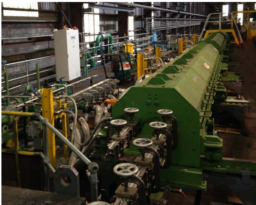
Figure 4 – Water box area after modernization
