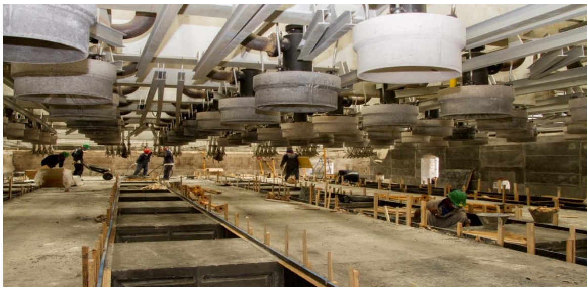
Figure 2: Internal view of the Billet Reheat Furnace during construction.
