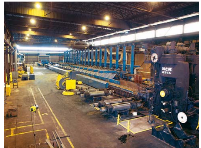
Figure 3 - View of the finishing area during the revamping
