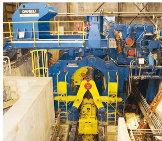
Figure 11 - The new downcoiler during the installation
