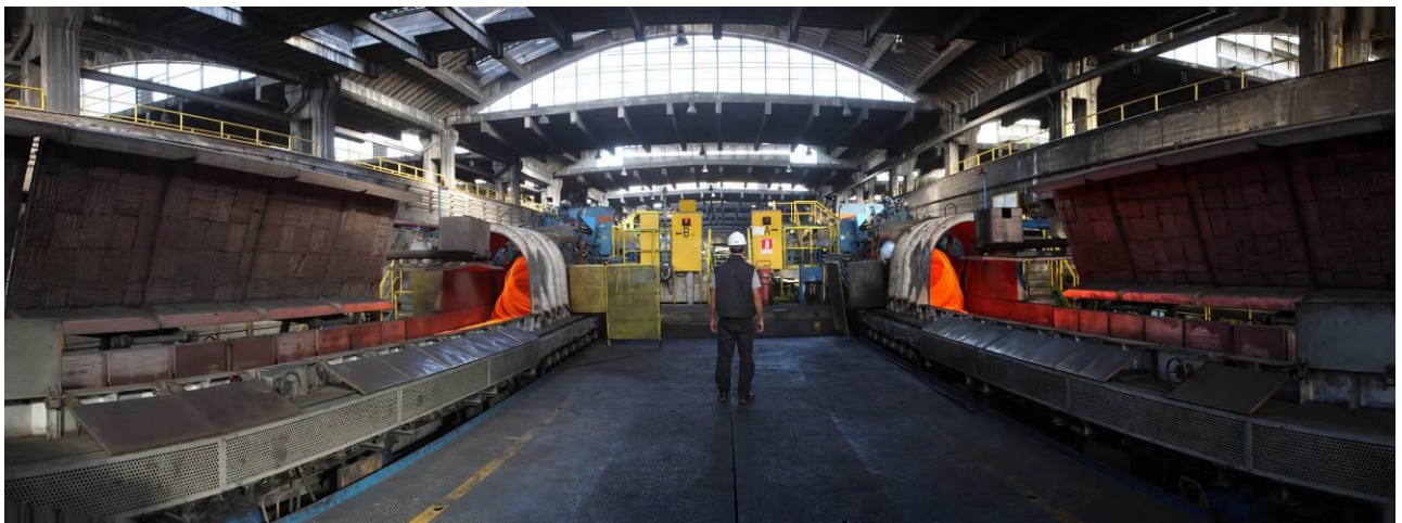
Figure 2. The latest generation OFB-LLH in operation at SN Longos – Portugal
