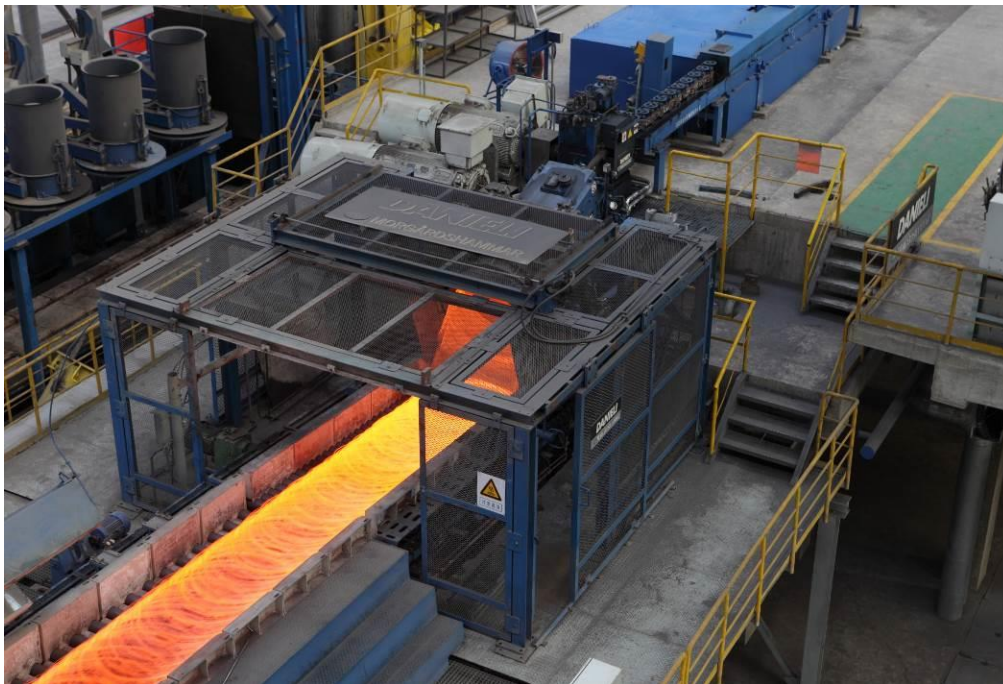
Figure 3. The latest generation LLH in operation at H 3 High-speed wire rod mill in Tianjin MGZY I&S – P.R. of China
