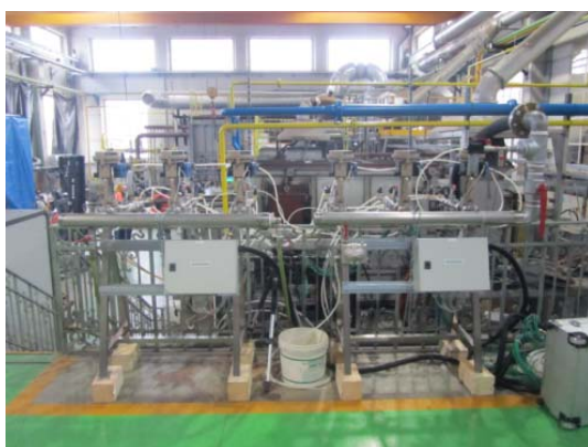
Figure 17 Pilot plant at RINA-CSM laboratory
