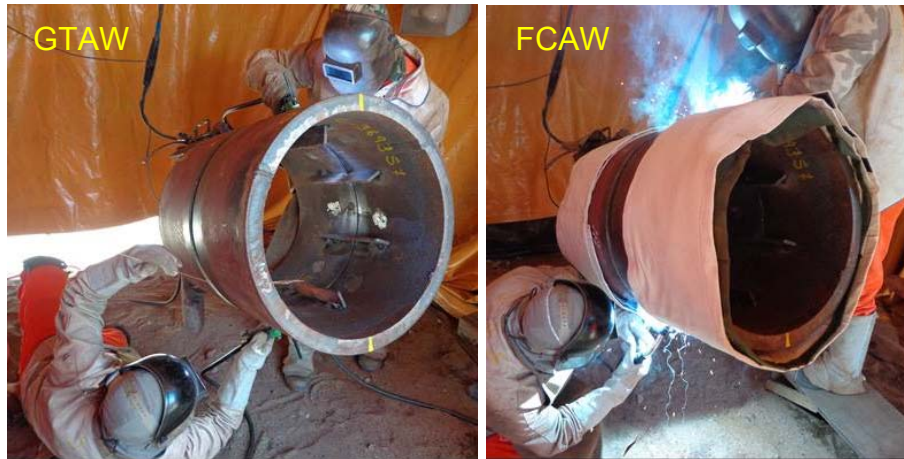
Figure 1. Welding of test joints.
