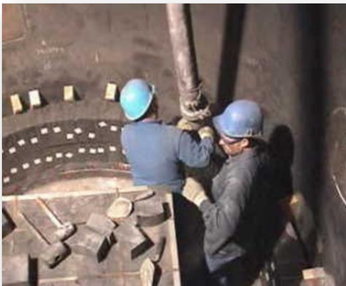
Fig.4: Casting behind the bricks
