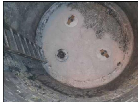
Fig.9: recasting of the bottom at the end of the campaign
