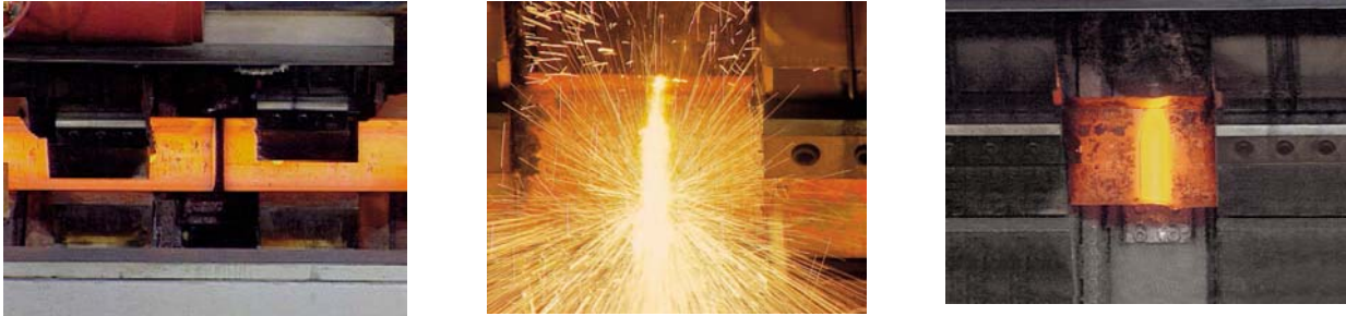
Pic 3 - Main steps of the welding sequence
