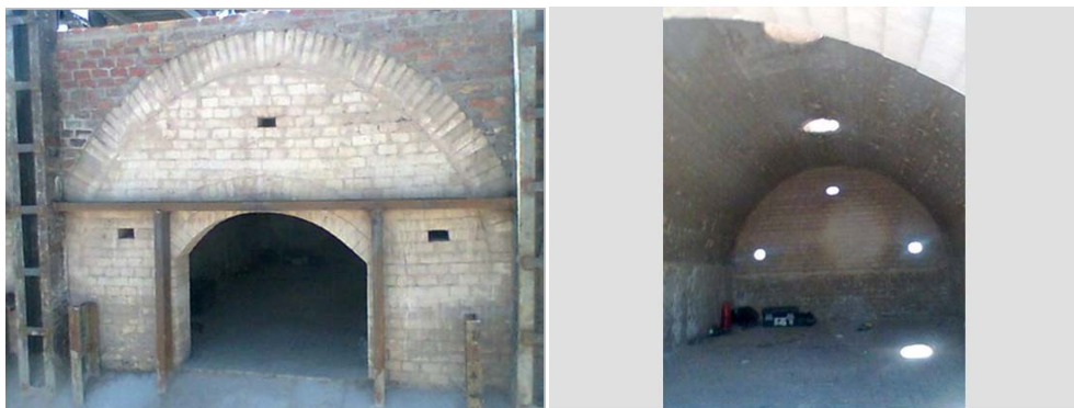
Figure 5. Typical non-recovery coke oven design [7].
