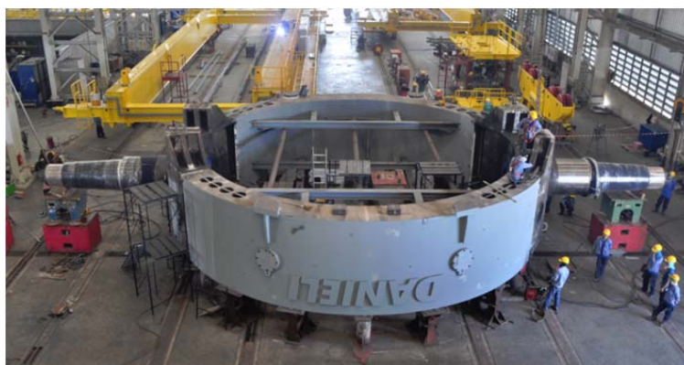
Figure 12. Final fit-up of trunnion ring in workshop before shipment.
