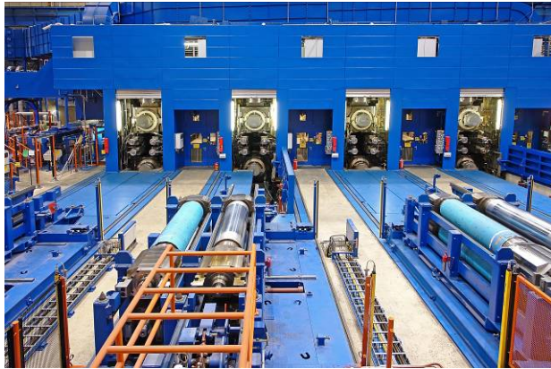
Figure 12: TCM, voestalpine, Austria
