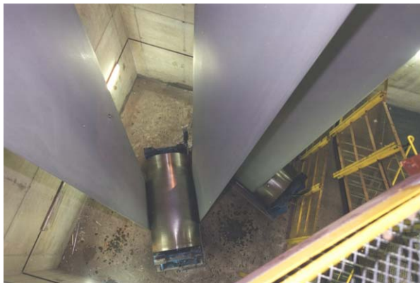
Figure 5: Arcelor Mardyck – turning tower
