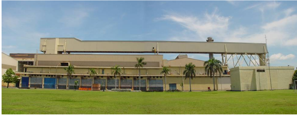
Figure 7: Krakatau Steel – looper on the roof
