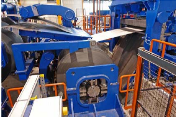
Figure 18: voestalpine Stahl - coiler
