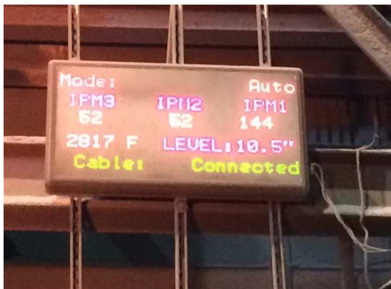
Fig. 13 LED Display Casting Bay
