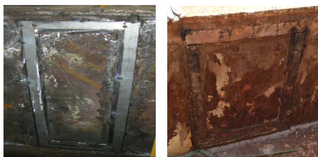
Fig. 6 Sensor Loop Installation
