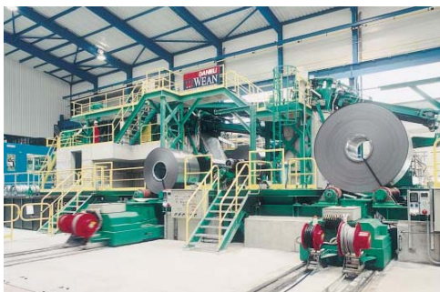
Figure 3. Overall view of the entry section.
