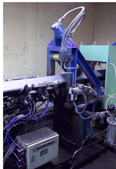
Figure 3. UT inspection station
