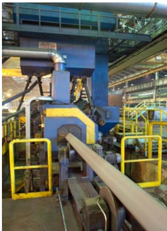
Figure 2. Shot blasting, cleaning unit
