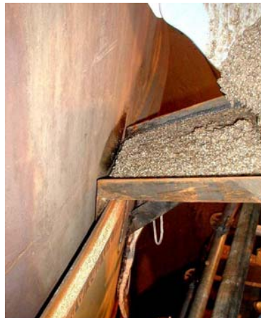
Figure 9: Casting of Epoxy Resin Stellatar to Protect Horizontal Weld
