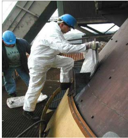
Figure 10: Filling of Dry Castable Carsit into Double Shell Gap
