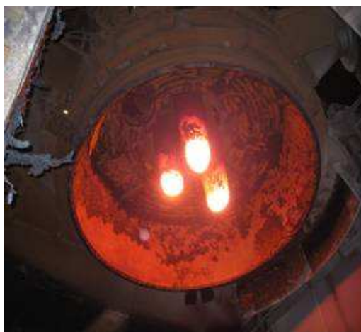
Figure 6. LMF copper roof.
