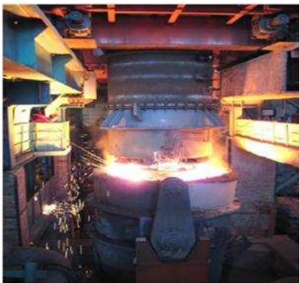
Figure 7. RH Plant at ZHF.
