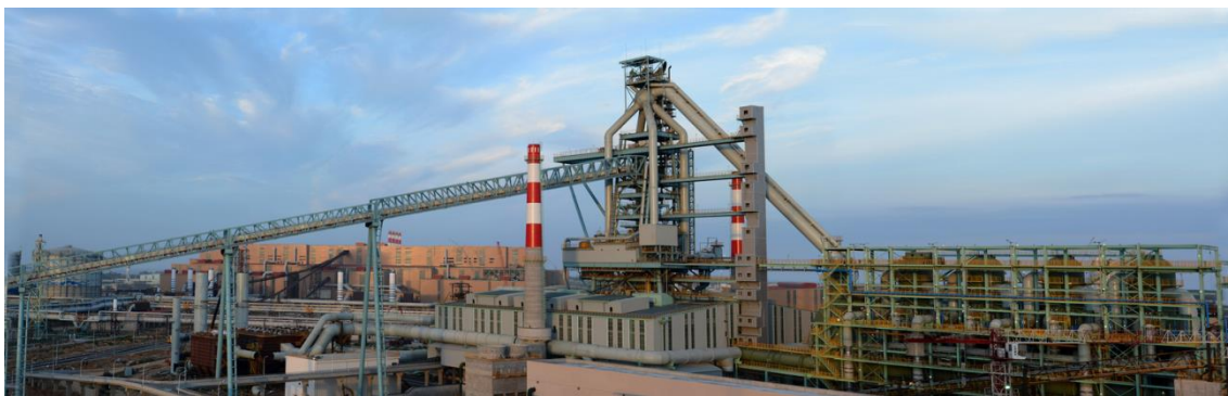
Figure 1 Picture of Zhanjiang No.1 BF
