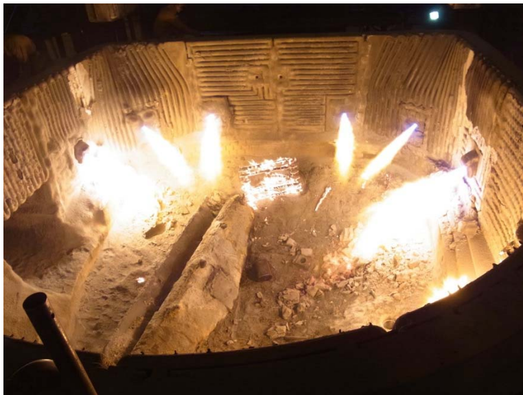
Figure 10: Interior view of the Finger Shaft furnace at Stahl Gerlafingen with installed tiltable VLB
