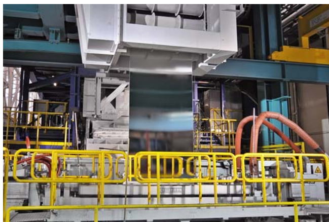
Figure 13: Zinc coating area.
