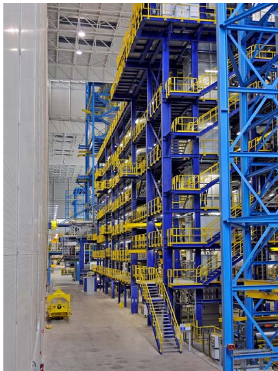
Figure 7: Furnace CGL no. 5.
