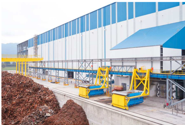
Figure 3. Loading hoppers at the scrap yard
