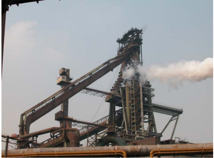
Figure 9 - Baosteel No. 3 Blast Furnace
