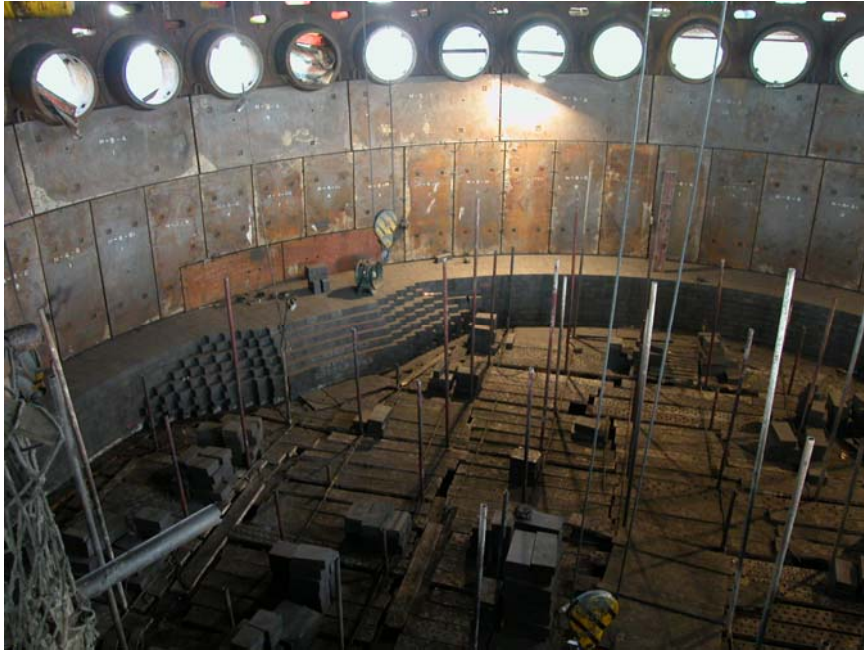
Figure 10 - Installation of the UCAR lining in Baosteel No. 4 Blast Furnace
