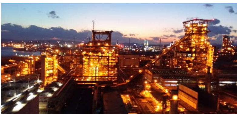
Figure 5: FINEX ® F-2.5M Plant
