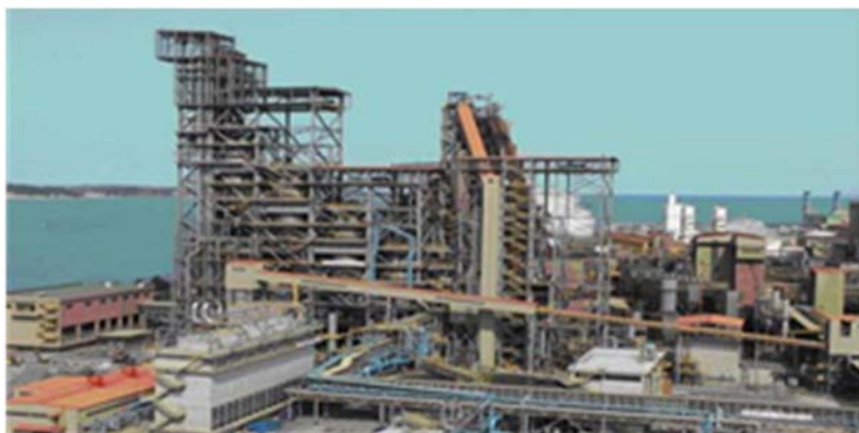
Figure 4: FINEX ® F-1.5M Plant
