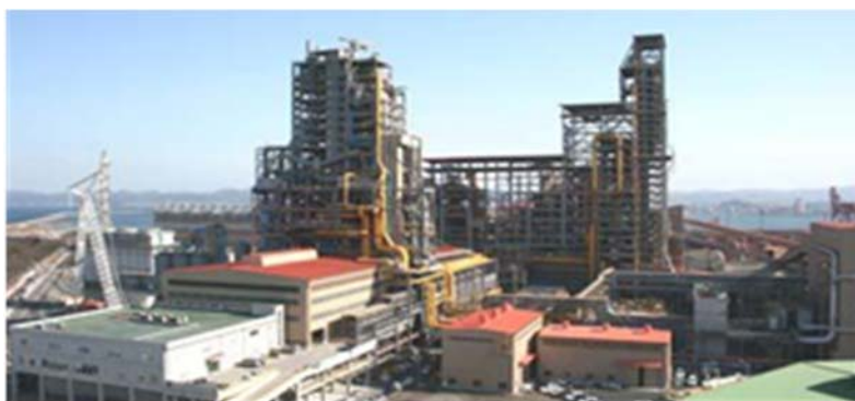
Figure 3: FINEX ® F-0.6M Demonstration Plant
