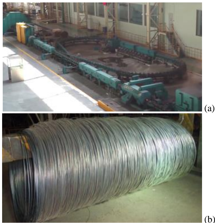
Figure 7. (a) Waterboxes installed in loop configuration in PFB area, (b) “Red rust” on \text{Ø}5.5\text{mm} 72D2: effect of different LLH temperatures on the same billet
