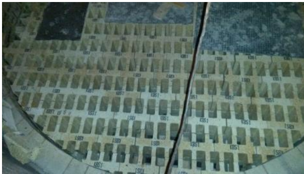
Fig. 10 – Burner after repair
