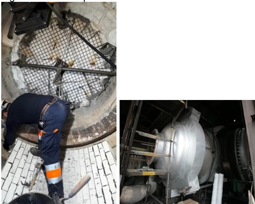
Fig. 7 – Hot blast main end cover during repair vs. end result
