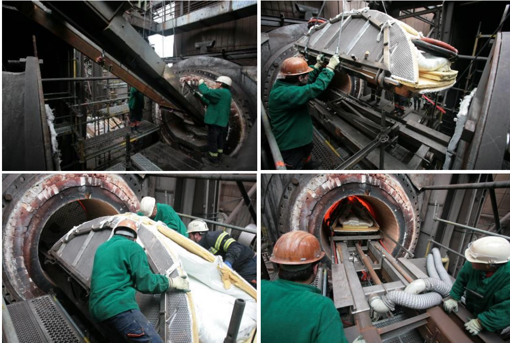
Fig. 8 – Installation of the heat shield
