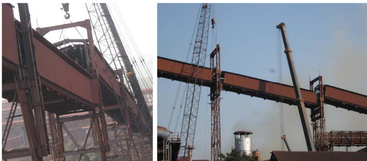
Figure 6. Lifting of main charging conveyor
