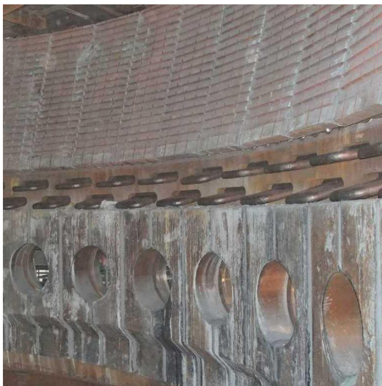
Fig. 4 Tuyère staves, cooling boxes and bosh staves during before refractory installation
