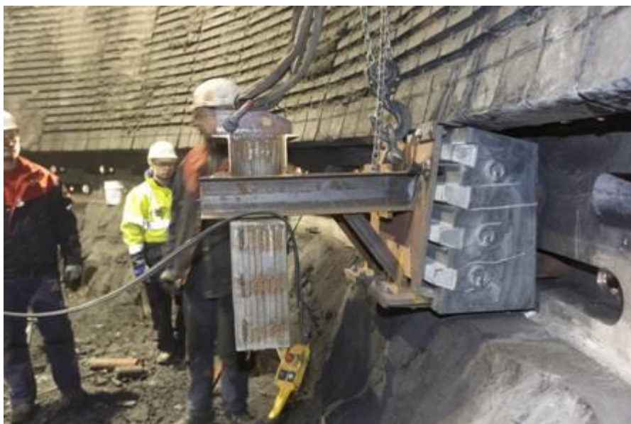
Fig. 10 Installation of the new copper staves between tuyère stave and bosh
