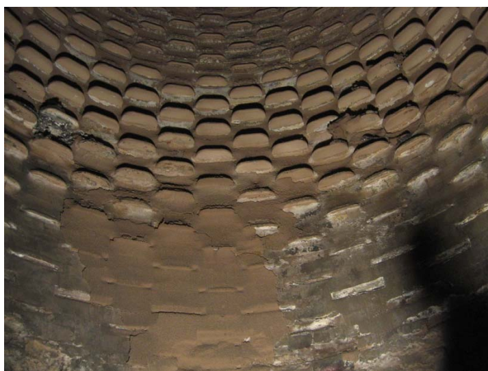
Figure 5. Furnace internal condition in 2006.
