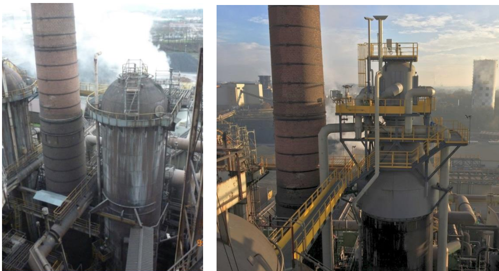
Fig. 9: Stove 15 before and after installation of the Paul Wurth DCS Burner
