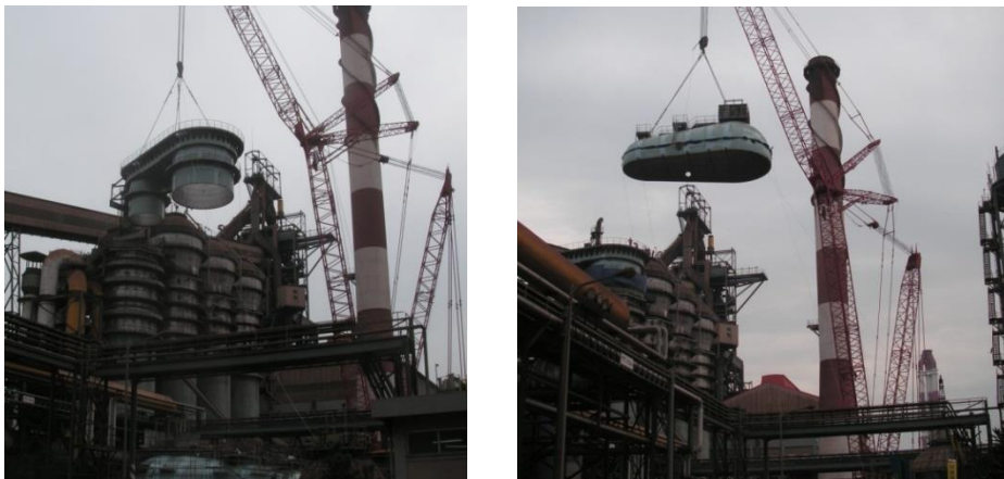
Fig. 7: Lifting of pre-fabricated dome into position during a dome replacement repair
