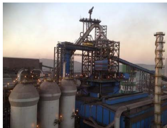
Figure 8. Blast Furnace amidst existing plants
