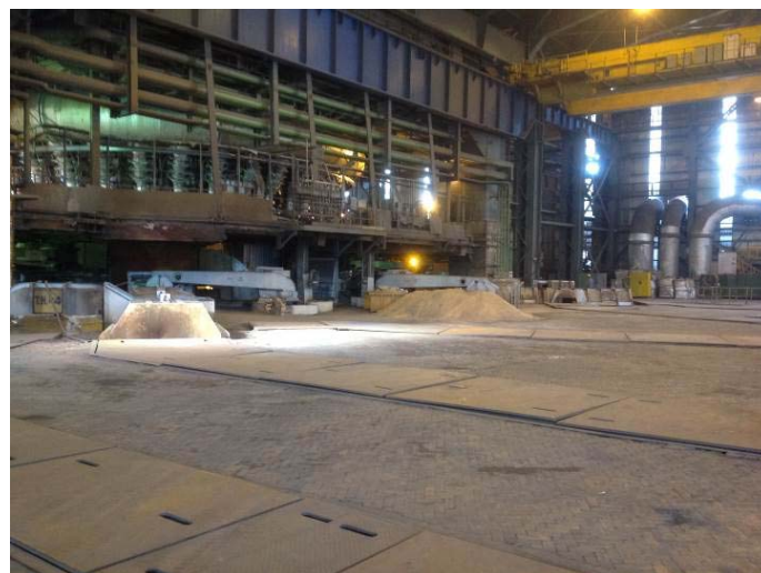
Figure 10. Flat Casthouse Floor
