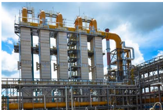
Figure 7 PT. Krakatau-POSCO Coke Oven Plant and By-products
